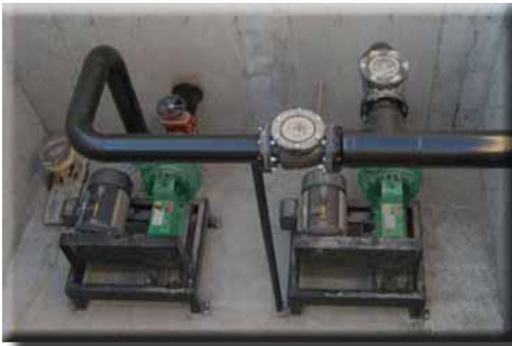
Separator feed pump in drywell for lower horsepower usage and longer life expectancy. Using GreenLine 8X6X14 pumps.
