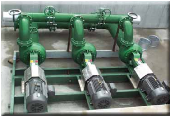
GreenLine 10X8X14 Flush pumps for two 7,000 cow dairies with back-up pump.
