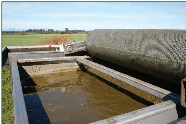
Built in bypass
